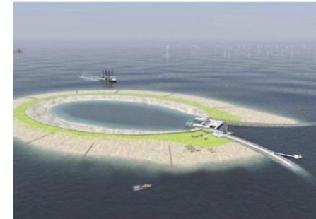
This illustration shows how the artificial island would use pumped hydro energy storage where water is pumped to a reservoir during off-peak times and released to a lower reservoir later to generate electricity.
